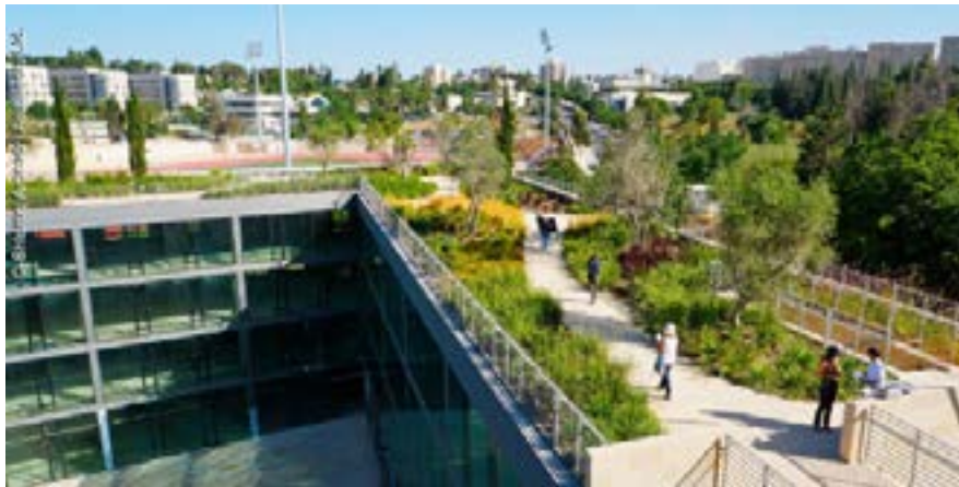
Figura 5. Cubierta intensiva con arborización. National Campus for the Archeology of Israel. Fuente: Shlomo Aronson Architects Ltd. (National Campus for the Archeology of Israel, Jerusalem | ZinCo Green Roof Systems, s. f.)
